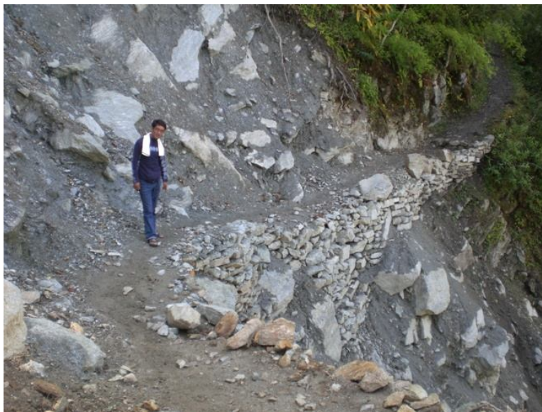
The way has been reconstructed stone by stone
